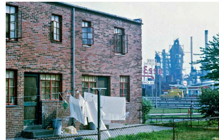
1986 - Philadelphia, PA. Project next to the freeway and ESSO oil refinery
